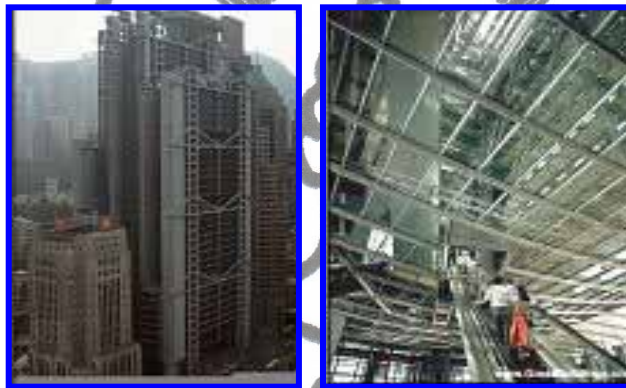
Gambar 2.14 Hongkong and Shanghai Bank Sumber: www.greatbuildings.com .
