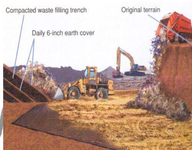
Gambar 2.2 Sistem Sanitary Landfill
