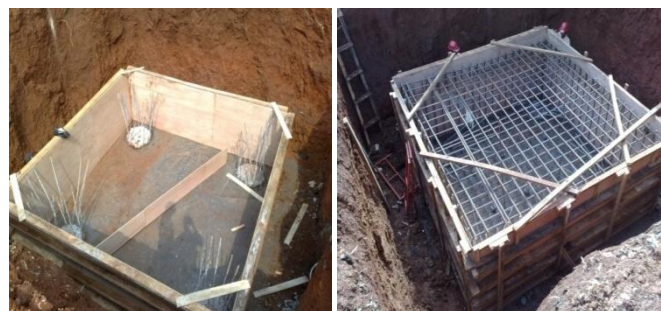
Gambar 4. Pondasi Tower Crane Sumber : PT. Tatamulia Nusantara Indah, 2010.
