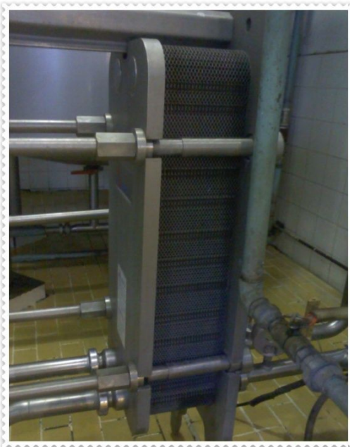
Gambar 4.10 PHE (Plate Heater)
