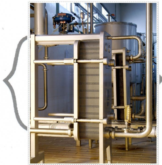
Gambar 4.4 Plate Cooler
