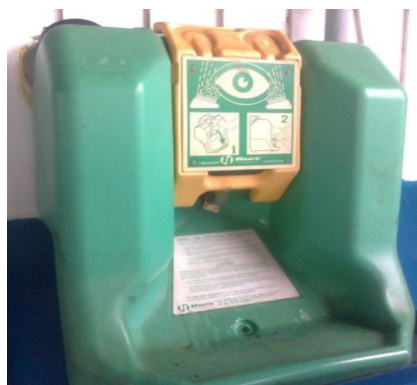
Gambar 13. Eye Wash Station
