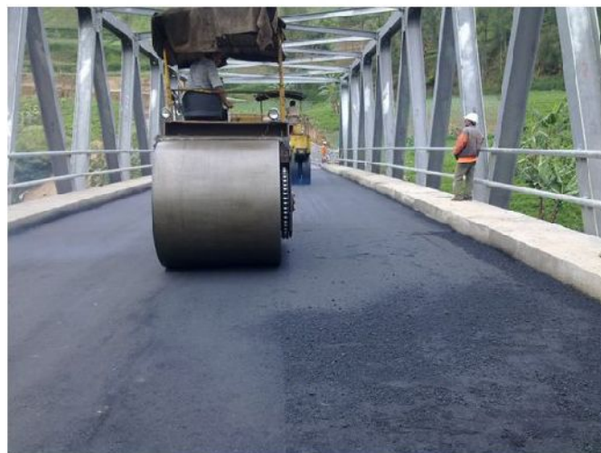
Gambar 4.6 Tandem Roller
