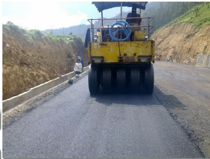
Gambar 4.7 Tire Roller
