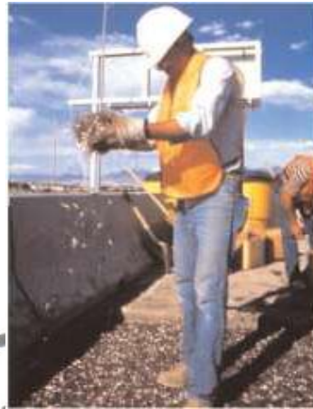
Figure 2.7 Tightly bunched steel fibers are placed in a form, before cement slurry is poured into this application of slurry-infiltrated steel-fiber concrete (SIFCON).
