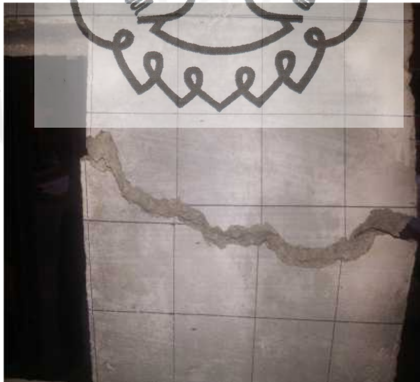
crack pattern under axial load
