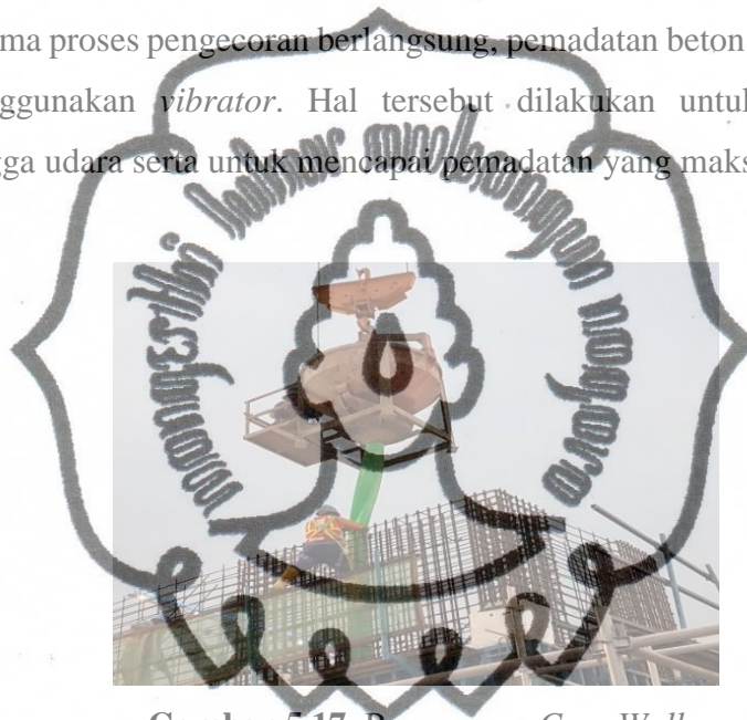
Gambar 5.17. Pengecoran Core Wall
